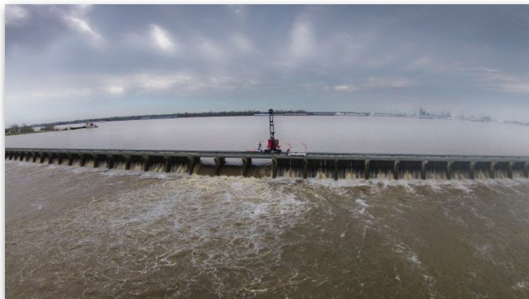
Bonnet Carret Spillway floodwaters release.
